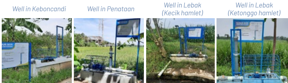
Four constructed wells in Kebon Candi, Lebak (Ketonggo dan Kecik hamlets) and Penataan villages
