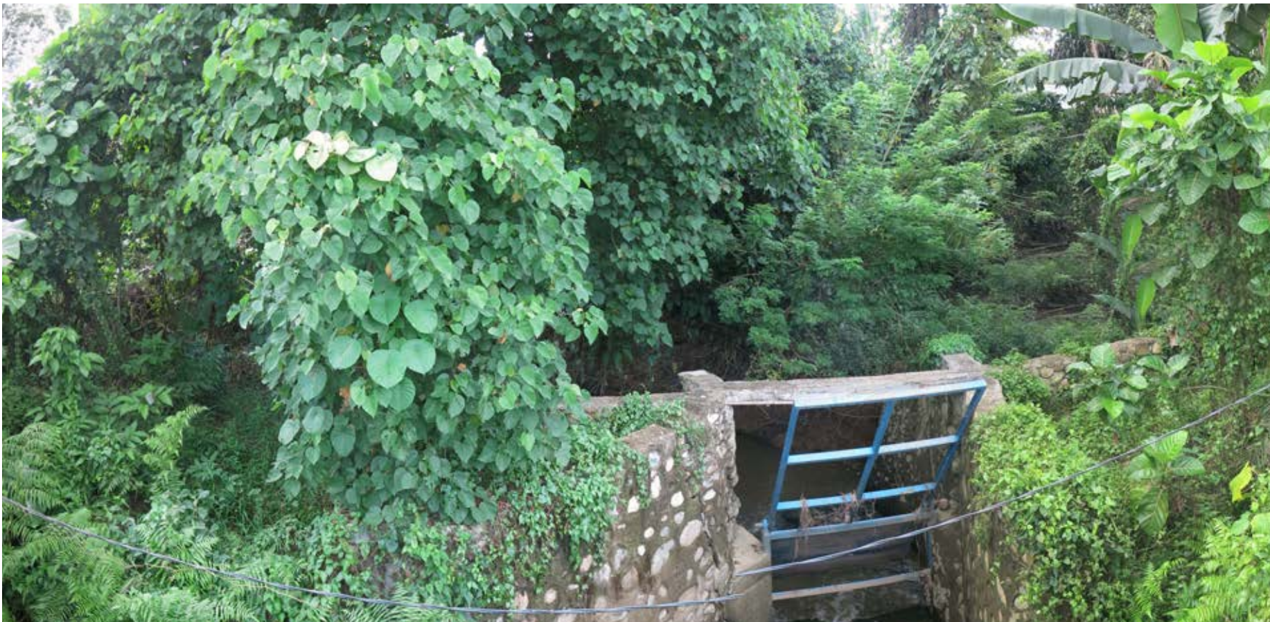
The sluice should have used a valve - This water sluice is supposed to automatically close when the water rises from the river. In reality, it has never functioned since it was built. I don't know what the mistake is. It needs to be rebuilt. Repairing is not the solution. We have to rebuild it from zero. (a male smallholder from Air Terang Village)
