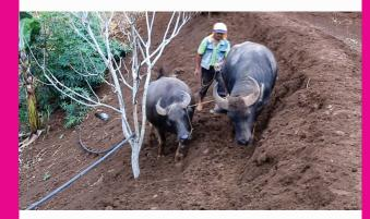
The tools needed to construct an animalbuilt embankment are generally available in any local farmers' arsenal. ABE makes use of wooden animal-drawn scrapers (ADS) instead of other mechanical tools.
