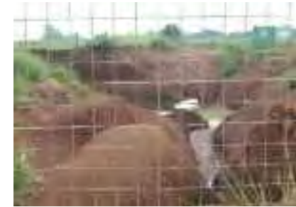
Fencing off and revegetating a 'donga' or eroding ditch
