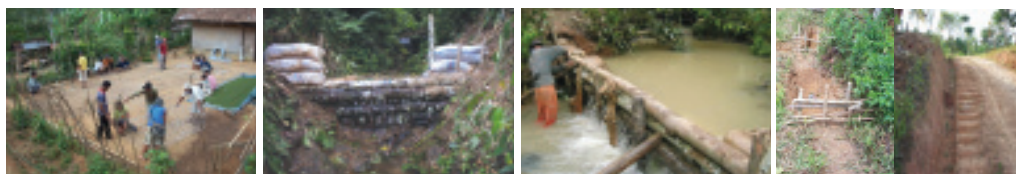
Community action: reduce runoff speed and trap sediment on path road (Photo credits: RUPES Sumberjaya Team)
