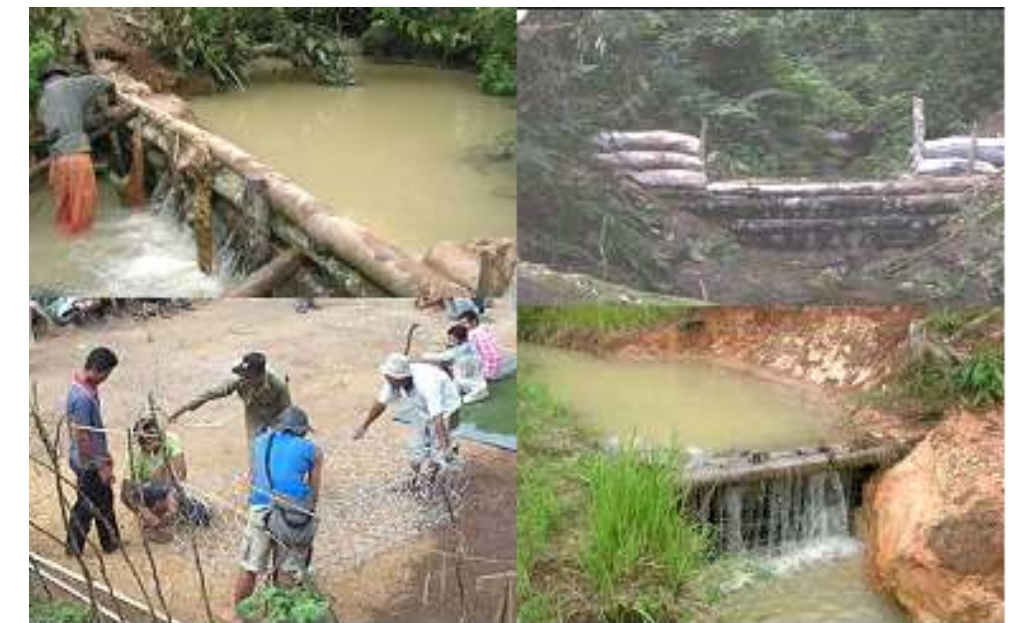
RiverCare: interventions to stabilize river channel and reduce sediment loads
