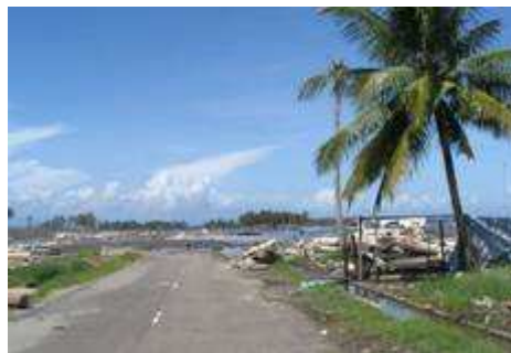
Figure 5. Reconstruction of washed away roads and bridges along the western coast of Aceh are vital physical capitals for post-tsunami recovery and future prosperity.
