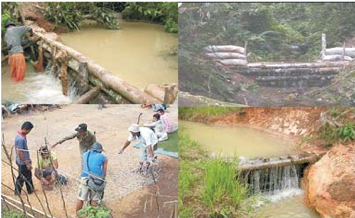
Community Actions: Control sedimentation and water flow from upper watershed, increase ground water table for surrounding areas.
