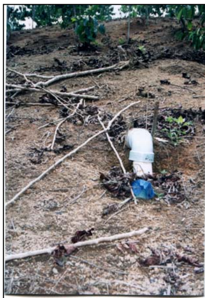
Figure 2.23. Litter of coffee leaves could change the direction of runoff and also block the collector of sediment trap
