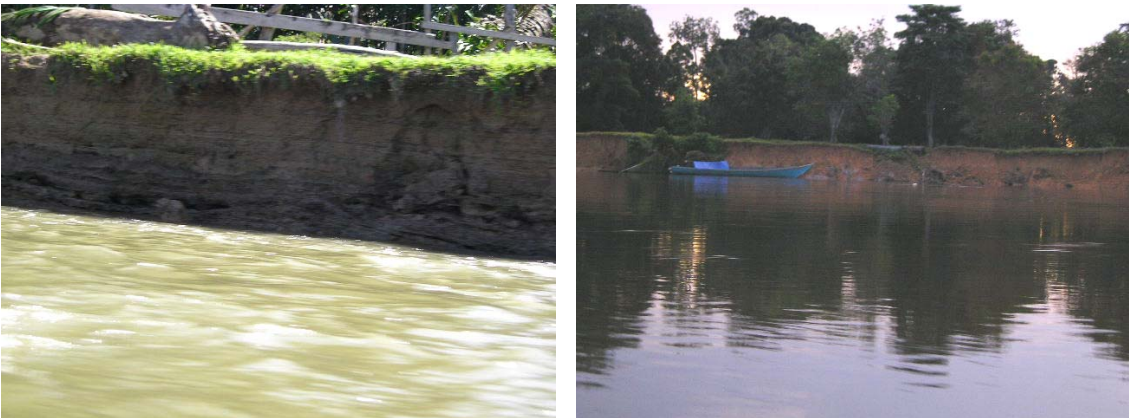
Figure 1 River bank collapse along the river in Kapuas (left) and Sibau (right)
